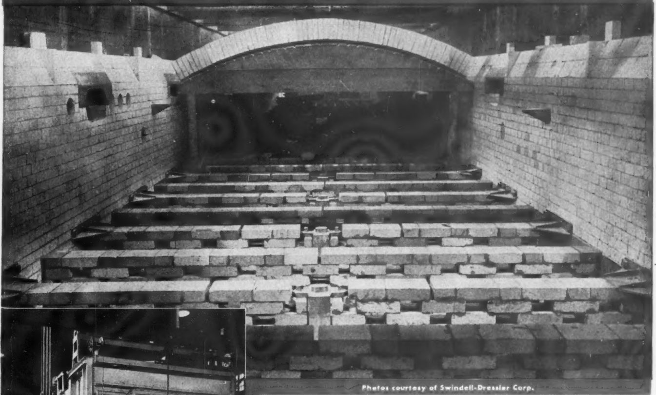
Photos courtesy of Swindell-Dressler Corp.
